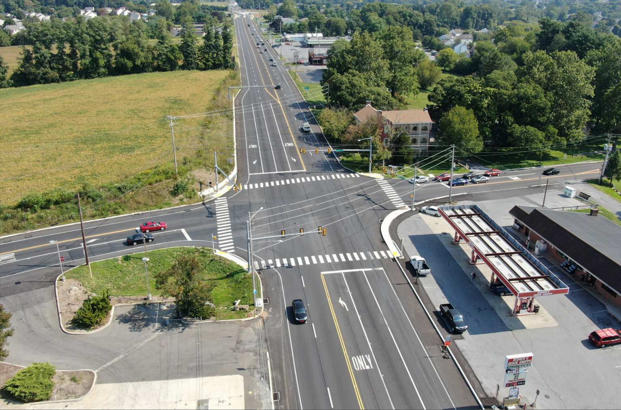
SR 0222 at SR 0073 Intersection – looking Northbound Widened intersection, added turning lanes and provided pedestrian crossings – Improvements avoided historic parcel in top right quadrant of above photo.
