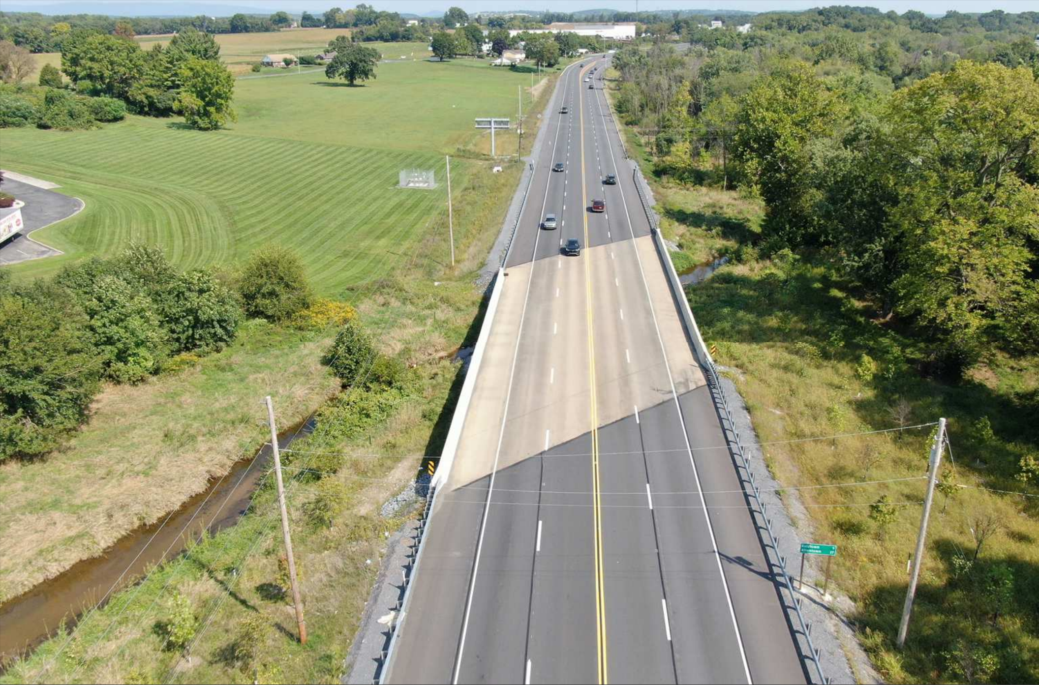
SR 0222 at Willow Creek Bridge – looking Northbound Four Lane Typical Section - relocated aerial poles and newly installed DMS sign along SB side of Roadway.
