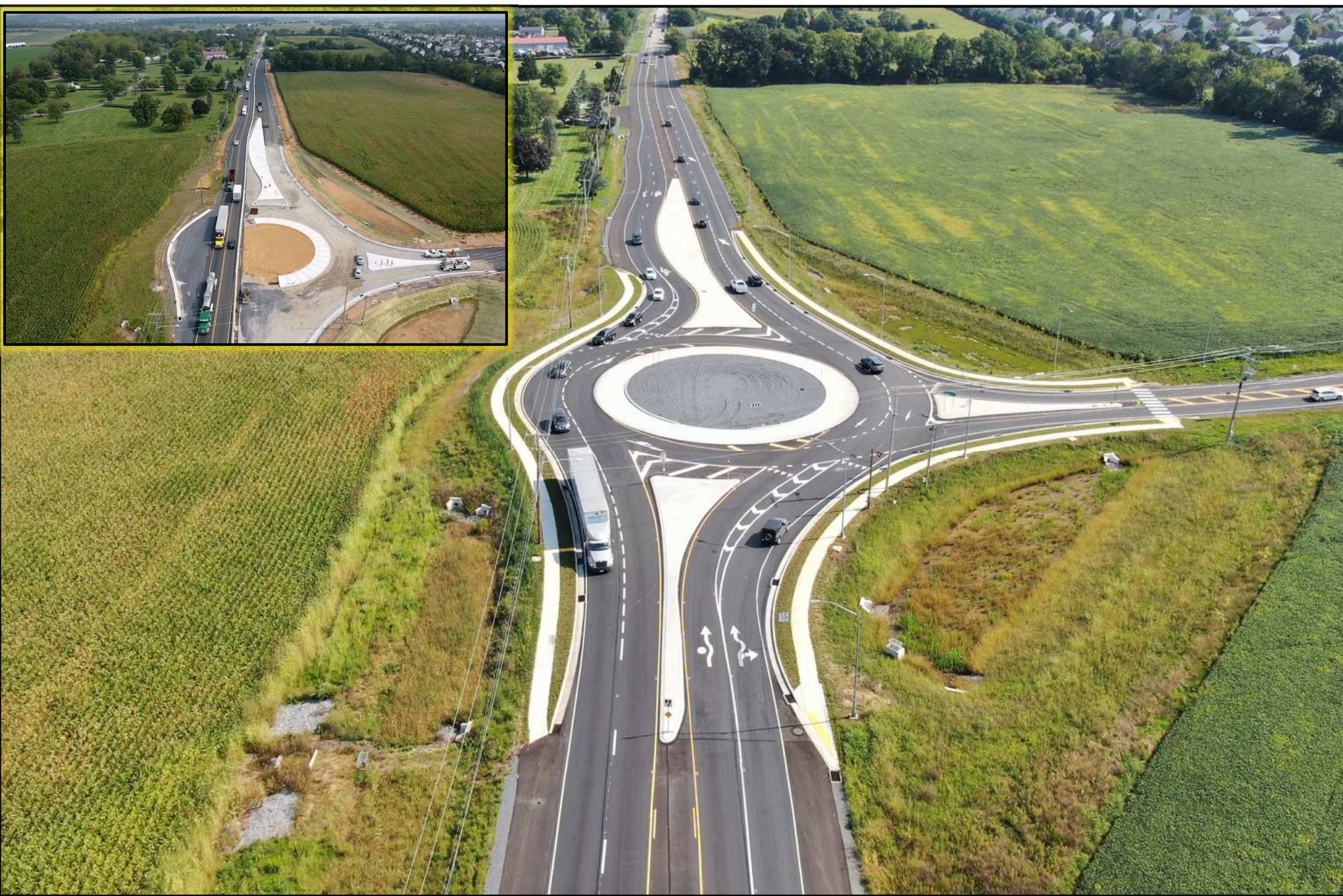
SR 0222 & Schaeffer Road Roundabout – looking Northbound
